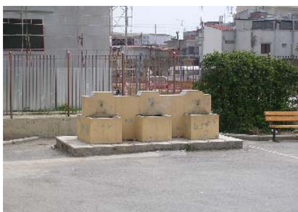
Evosmos: An example of the poor quality of existing facilities at a school in Evosmos
